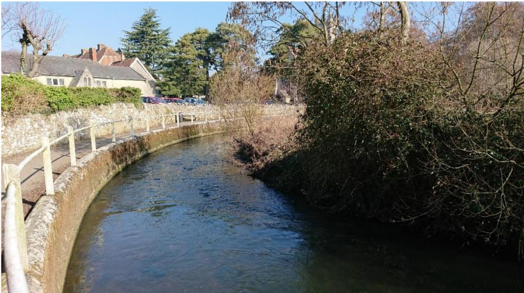
*Figure 3: Natural riffles towards the end of the reach visited. This figure also shows the concrete revetment.*
